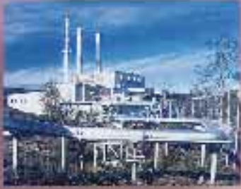
Iroquois Falls generating station, 110MW, 1996
