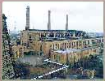
Darnytsia heat and power station, Kyiv, Ukraine 280MW
